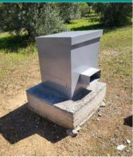
The RSD6000 can be housed in traffic cabinets, which are anchored to the sides of the road. This configuration requires an installation of the cabinets, but allows a fixed system to measure uninterruptedly, 24/7, at a specific site.
