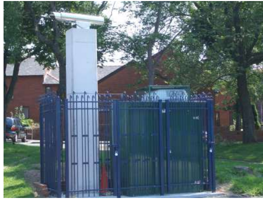
An Opsis open-path DOAS system in Swansea.
